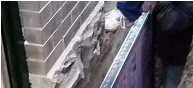
Figure 6. 2-inch rigid polystyrene below-grade perimeter insulation & drainage.
